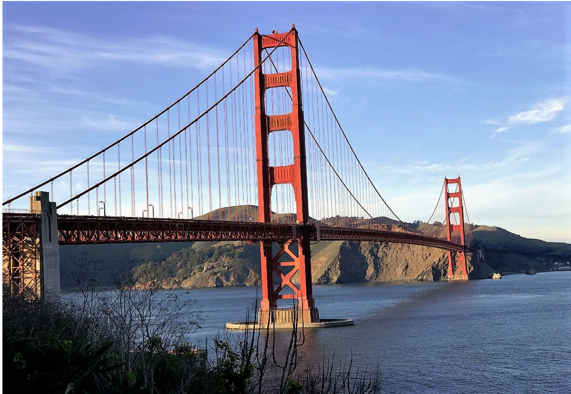
Golden Gate Bridge, San Francisco
